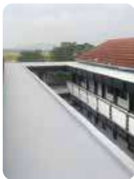
Shop building concrete deck
