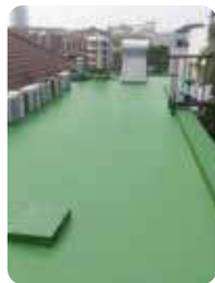
House & high rise building concrete deck
